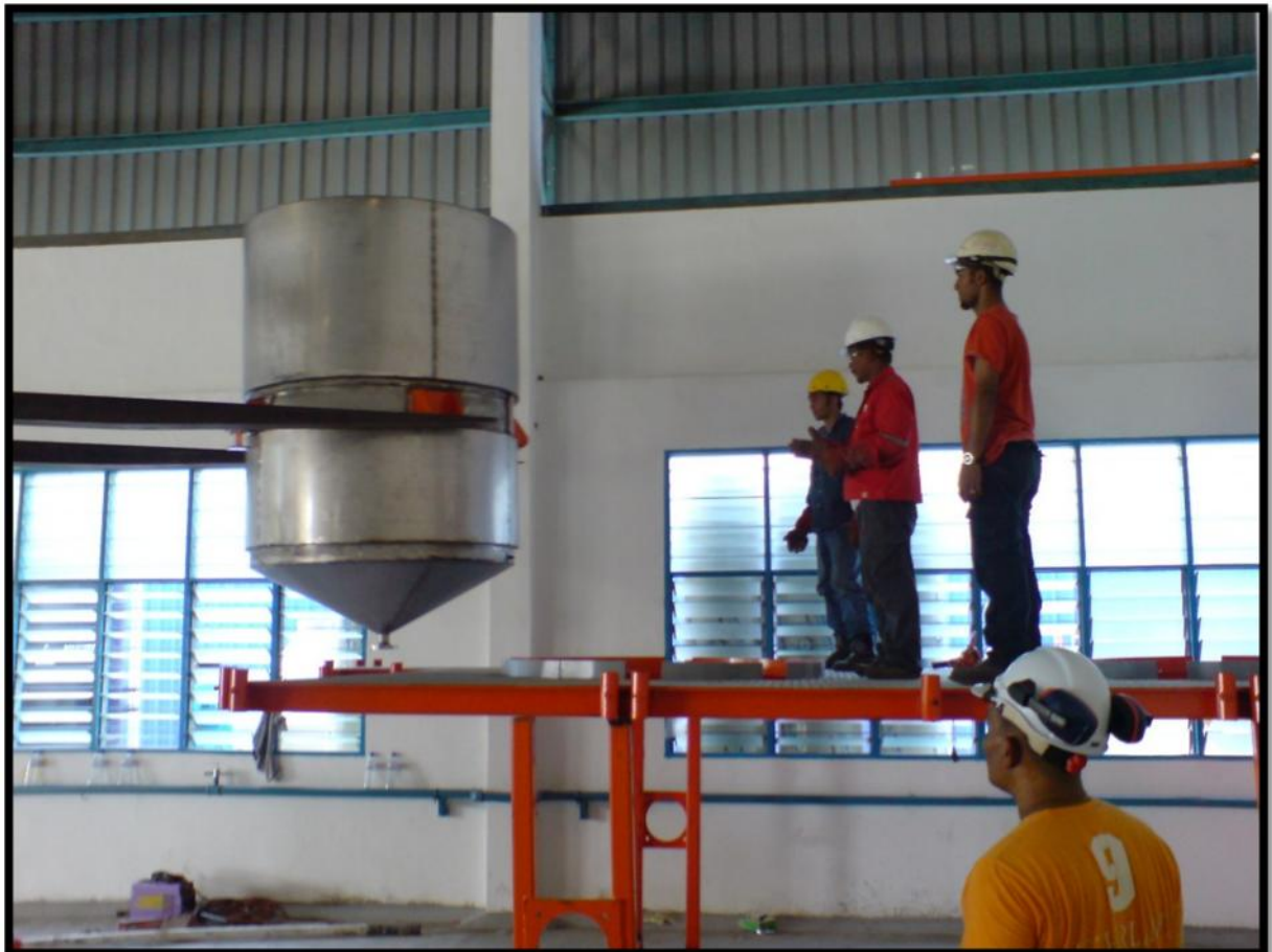
Plending tank & Platform for Clariant Oilfield at Pasir Gudang, Johor
