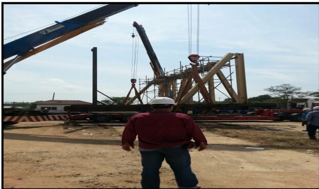
PHOTO: fabrication works for Tapis EOR Brownfield modifications and Retrofits projects.
