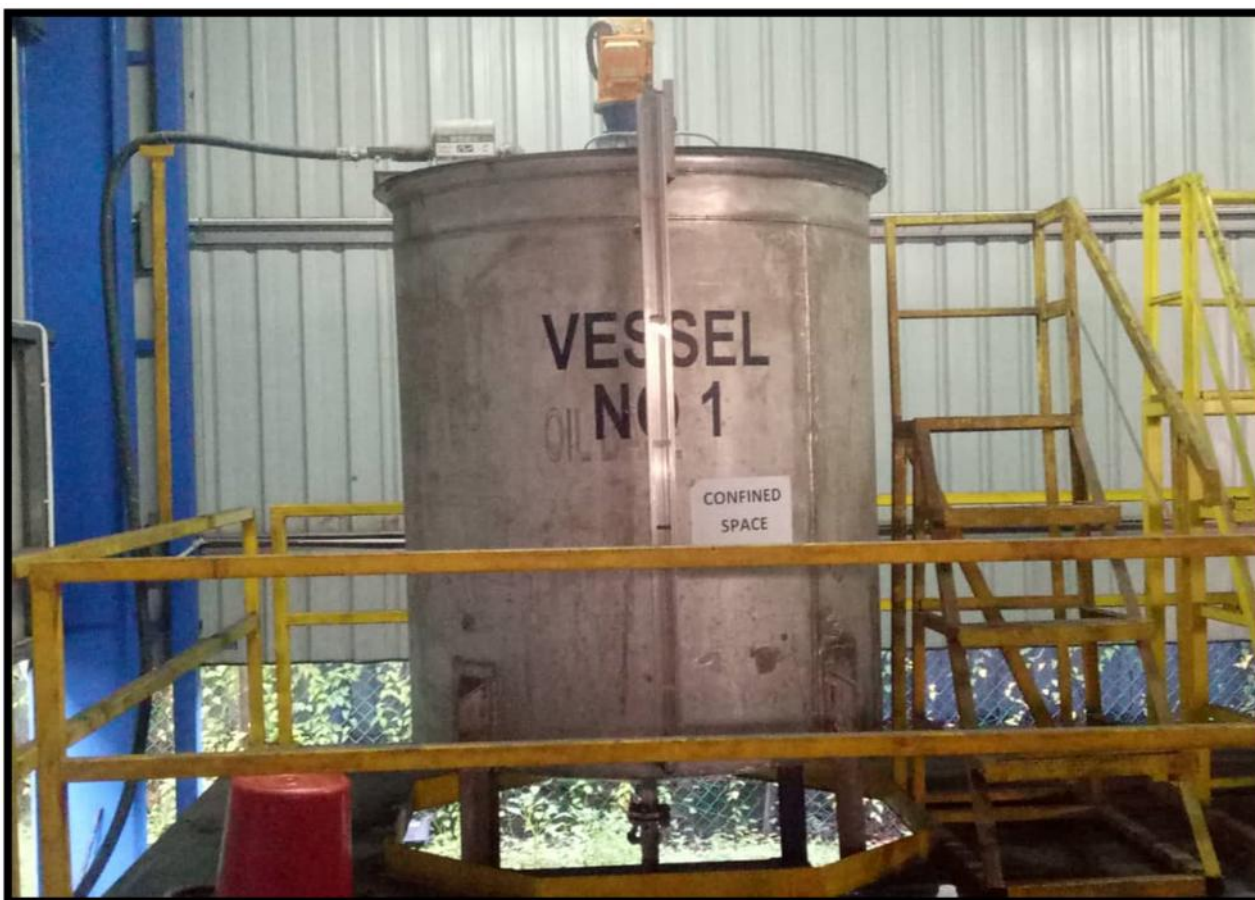
Blending tank & Platform for Clariant Oilfield at KSB Phase 2, Terengganu
